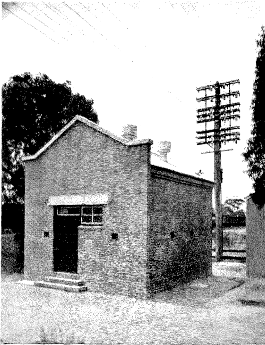
Fig. 14—Euroa repeater station.
